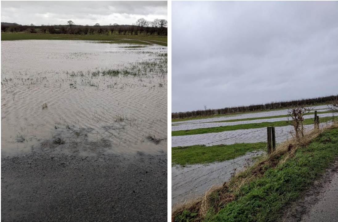
Flooding photographs adjacent to Burbage Common Road dated 2022, near to Woodhouse Farm Shop; this flooding is within the area intended for the employment units to be built
