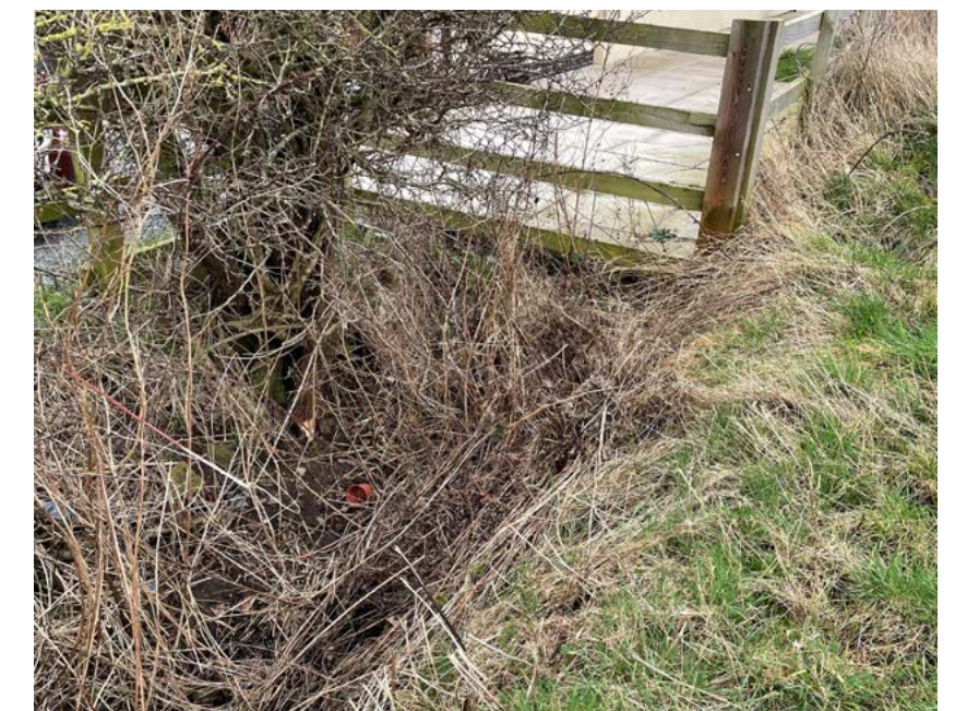
Existing culvert towards the north of the Site
