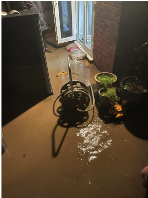
Pic. 4 Rear of 1 Station Road
