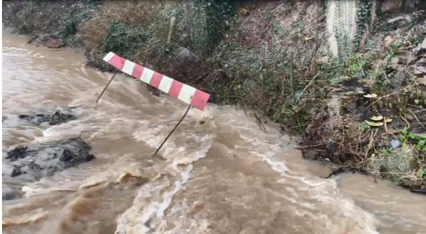
Pic. 9 Water Flowing into the restrictor plate overflow 14:02 2 nd January 2024
