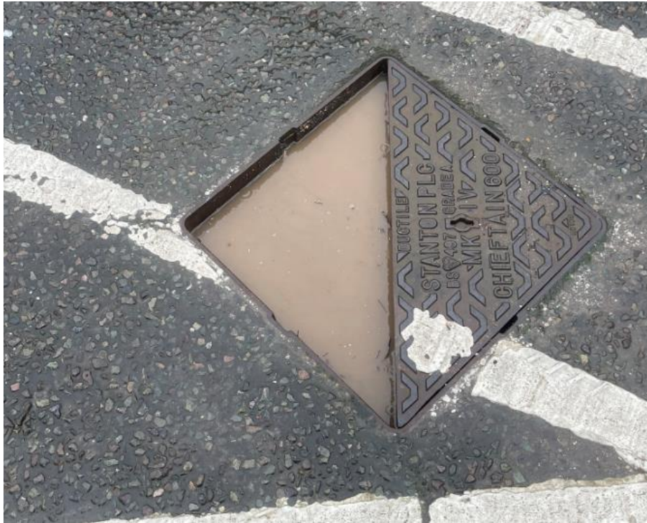
Pic.4 Manhole 5 at 13:02 2 nd January 2024
