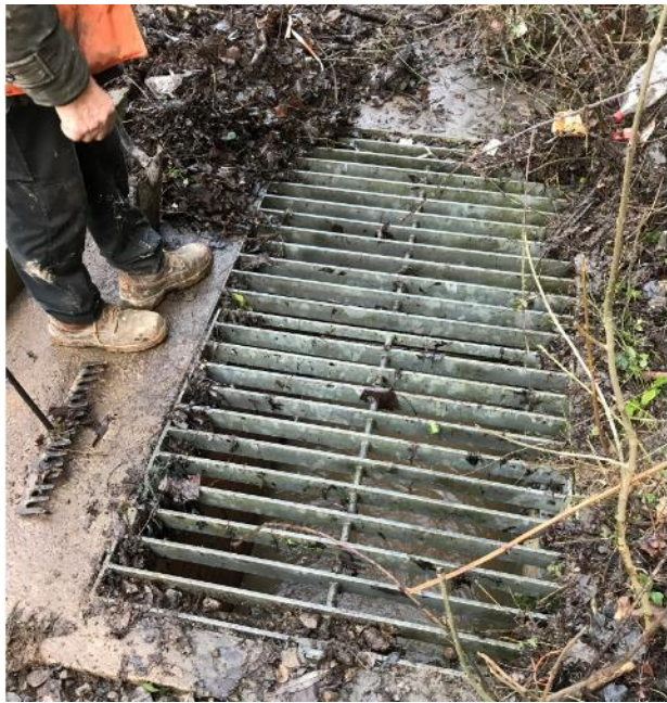
Pic. 11 Restrictor Overflow Grate post cleaning and water level receding.
