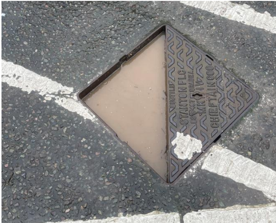
Pic.4 Manhole 5 at 13:02 2 nd January 2024
