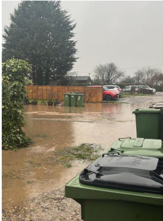
Pic. 14 Water accumulating to the rear of Station Road homes overspilling the bank of the brook and pooling in gardens 14:21 2 nd January 2024
