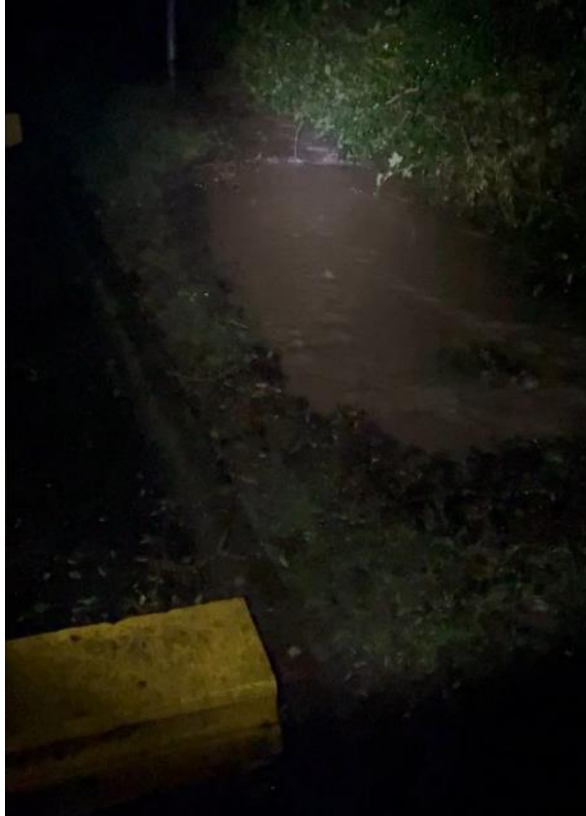
Pic. 8 Overflow from manhole 5 with no where for the water to go.
